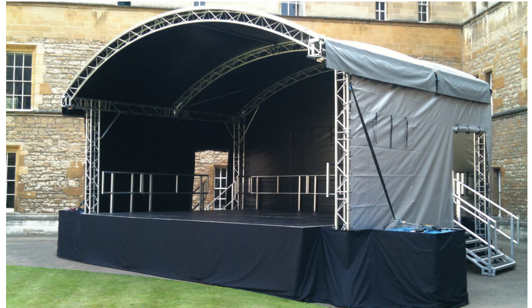
Private Event, Oxford (Structure with water ballast)
