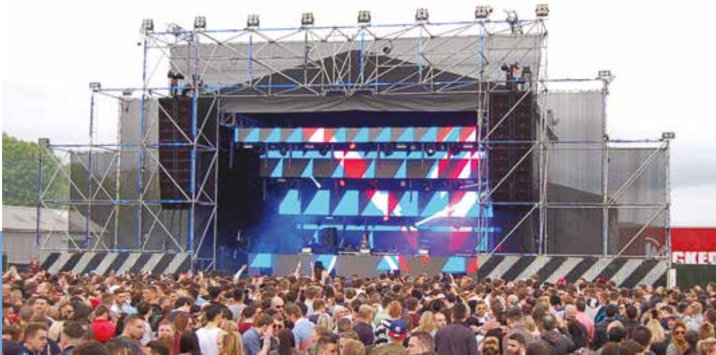
Shindig Weekender, Newcastle (Structure with Layher substructure and custom Layher Facade)
