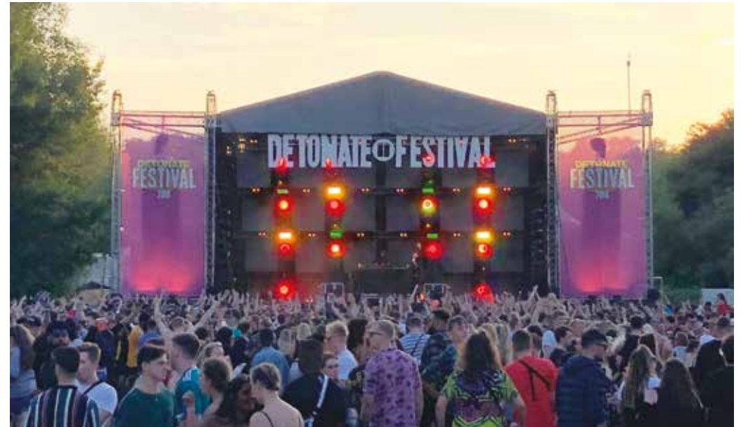
Detonate Festival, Nottingham (Structure on Layher substructure with Truss PA Wings)
